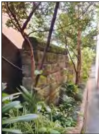
Existing remnant sandstone wall along the common side boundary of the subject site with 23 Billyard This wall is noted to be partially over the side of 23 (based on the survey). Potentially impacted by excavation, planting on the other side. Impact on this is not assessed in the documents.
